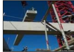
secondary beam installation
