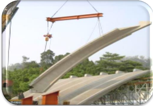
Prestressed Precast roof slab
