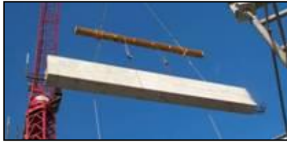
secondary beam installation
