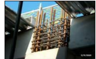
Reinforcement for Beam-column joint
