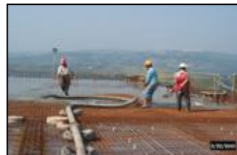
Reinforcement and concrete casting for floor
